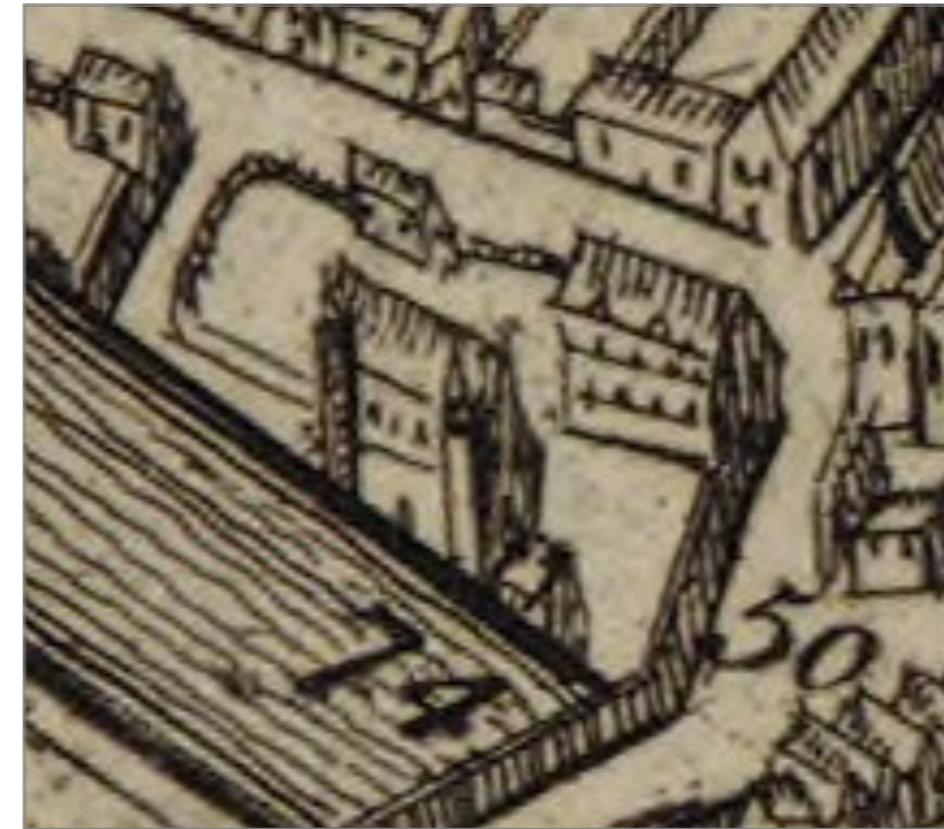
illustratie 82: Isaac Basire 1708 50= friars of y servants house 74 is Wieneraers brugge.
